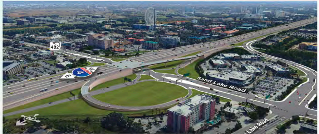
Sand Lake Road Interchange Improvements
